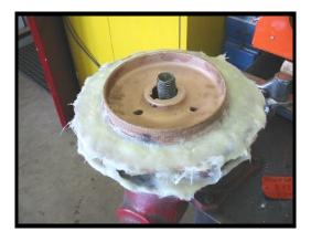
The impeller was then re-built using THISTLEBOND RESIN & HARDENER (TRK19000) plus THISTLEBOND FAIRING COMPOUND (TRK19042). This formed the bulk of the repair to recover lost material.
