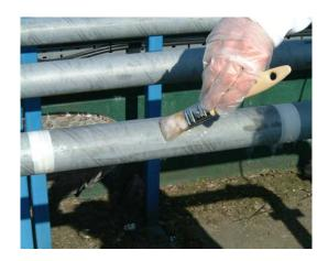
6. Thoroughly coat the surface of the repair area with the ThistleBond Standard Resin and Hardener mix.
