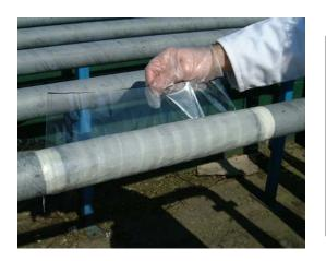
Cut a piece of Cellophane a little larger than the length of the repair and at least 100mm longer than the circumference. This is applied to the surface of the repair and should be retained in place by means of masking tape at each end of the repair.
