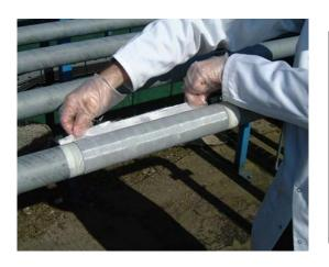
9. After the Glass Tape has been wound around the pipe work and the twice and third layer of Resin mix has been brushed onto the repair, cut a piece of Glass Cloth to a size that extends over 2" over the wraps of Glass Tape. Wrap the Glass Cloth over the pipe work
