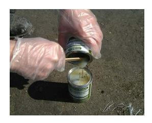
5. Mask off the section of pipe you wish to repair. Mix the tins of Resin and Hardener together, using the Wooden Stirring tools provided. Ensure that both parts are thoroughly mixed. NOTEusable life once mixed is 25mins at 20C
