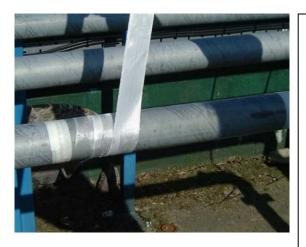
7. When Glass Tape is being used for the repair this should be wound round the pipe directly from the roll. The tape should be wound reasonably tight onto the Resin Mix coated surface of the repair to ensure the mix permeates through the interstices of the tape. The tape should be wound to overlap by half its width.
